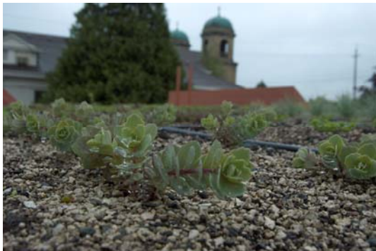
Green roof on new addition
