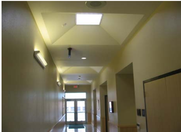
Hallways use skylights to bring in natural light
