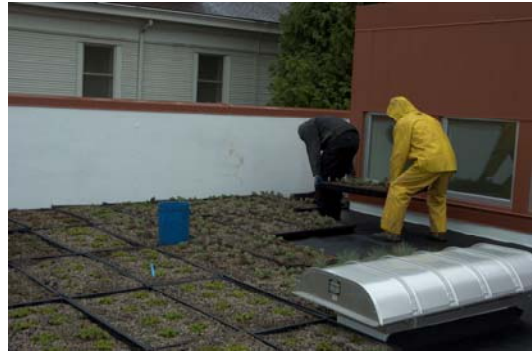
Workers installing GreenGrid
